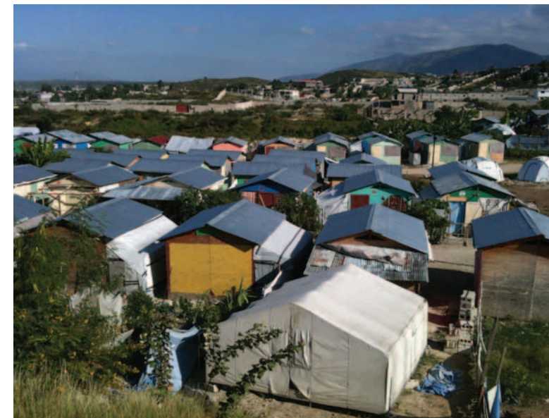
At Terrain Toto, CRS helped construct T-shelters in the camps. Photo by Seki Hirano/CRS.
