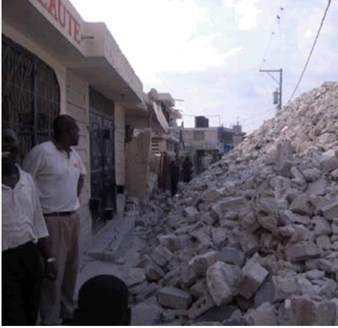
The scale of rubble in urban disasters can be huge. Photo © UN-HABITAT/Julius Mwelu
